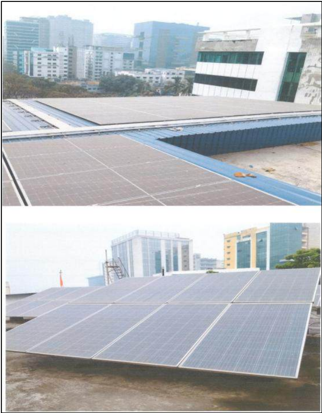
Roof-top Solar Panel
