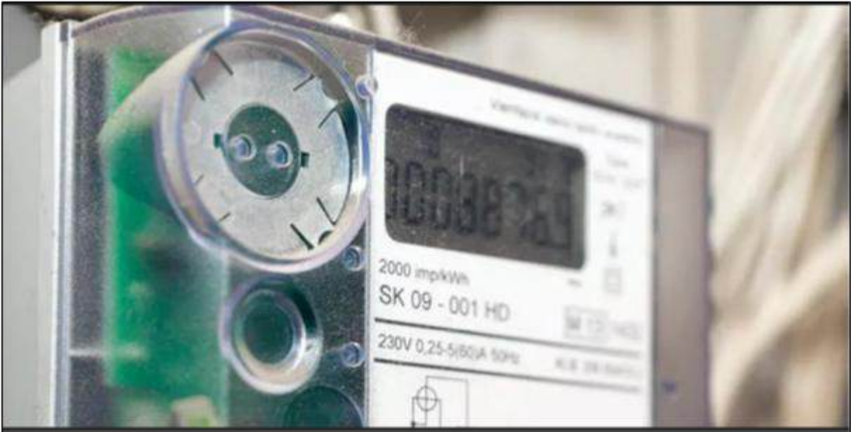
Installation of Smart Meters
