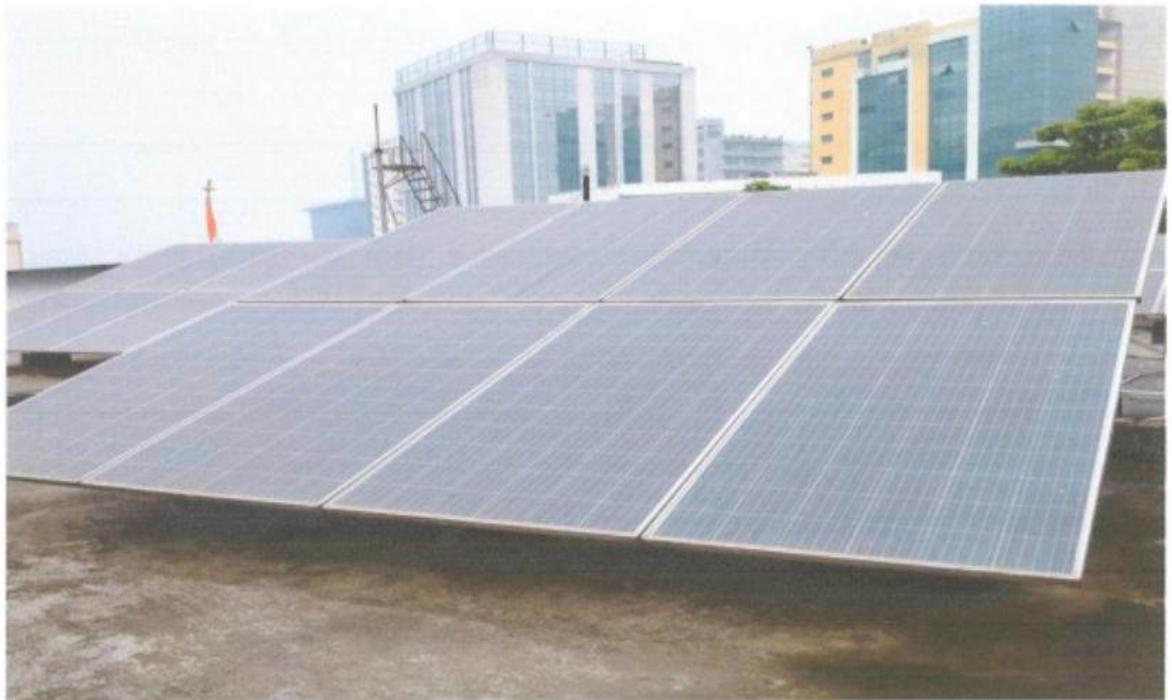
40 kW Grid-Connected Rooftop Solar Panels installed in IEM Newtown campus generating 320 kWh/day
