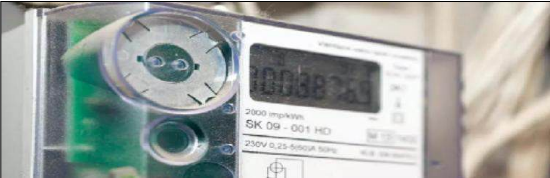
Installation of smart meters
